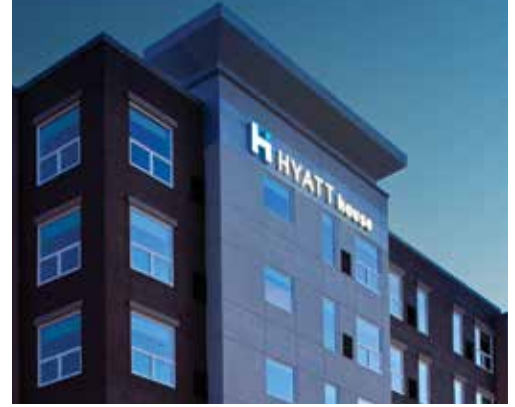
Hyatt House Denver/Lakewood at Belmar 135 guestrooms
